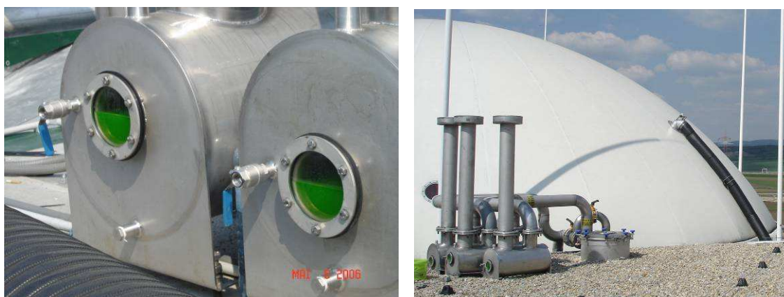
Figure 7.25 Safety pressure facilities and valves (AGRINZ 2006)
