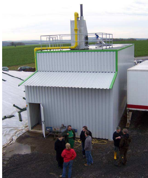
Figure 7.21 Horizontal plug-flow digester (RUTZ 2006)
