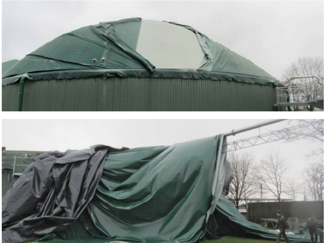
Example of a ripped gas storage
