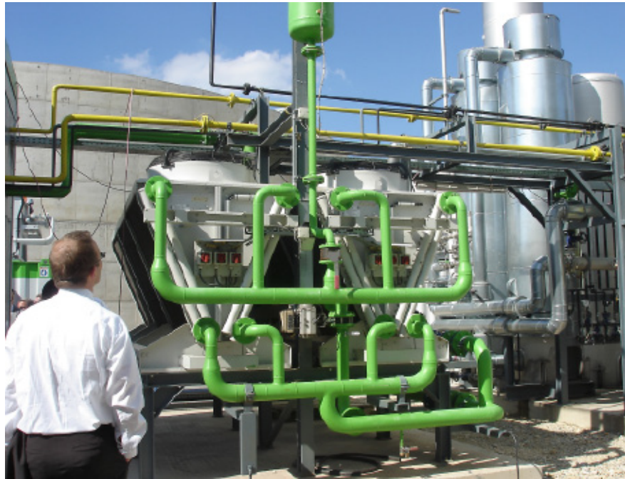
Biogas upgrading unit
