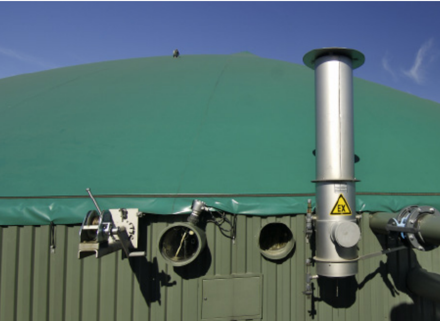
Overpressure and underpressure protection device on a digester
