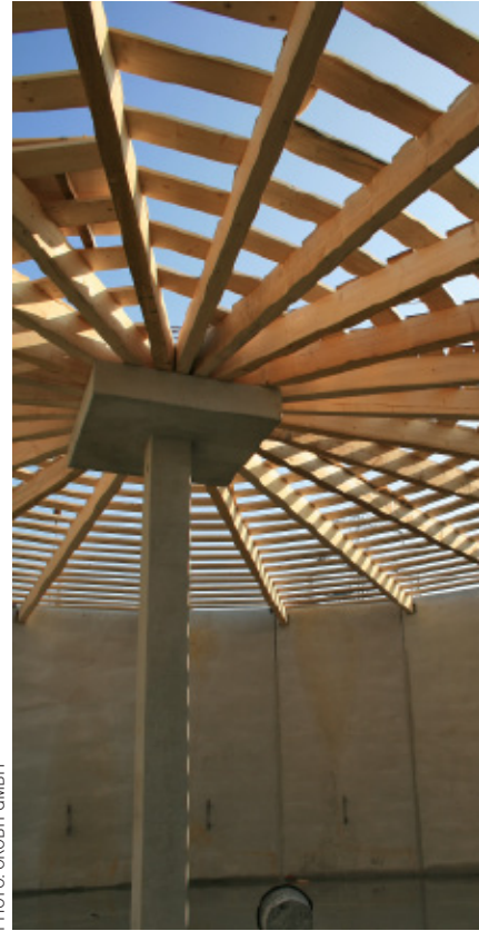
Wooden roof structure of a digester
